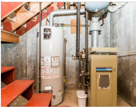
Hot water heater and furnace
