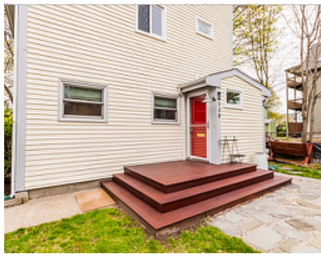
Exterior and entry
