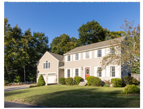
Introducing 5 Cornet Stetson Drive
