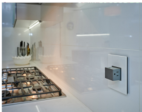
Kitchen – Retractable Outlets
