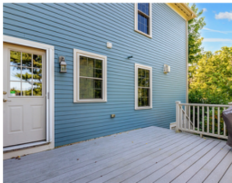
Deck— off kitchen
