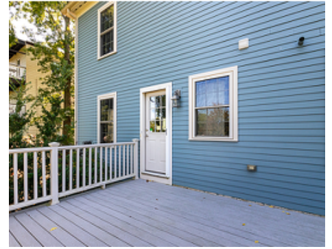
Deck— off kitchen
