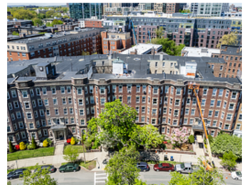
Aerial of building and block
