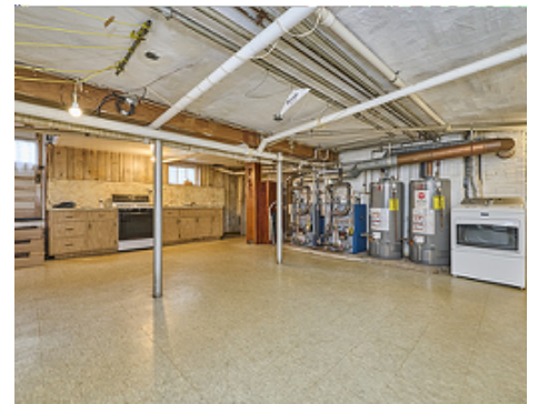
Kitchen / Utility Room
