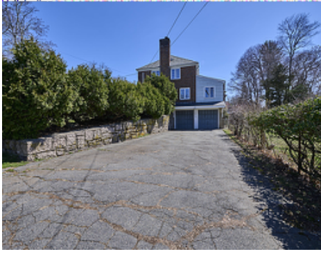
Side Garage View
