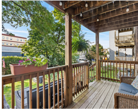
1st Floor Rear Porch
